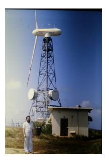
We visited a wind turbine site where we got wind blown and asked more hard questions such as why not use a lightweight alternator in the nacelle instead of a heavy, complicated AC synchronous generator. An inverter on the ground could handle several wind turbines and simplify both assembly and maintenance.
